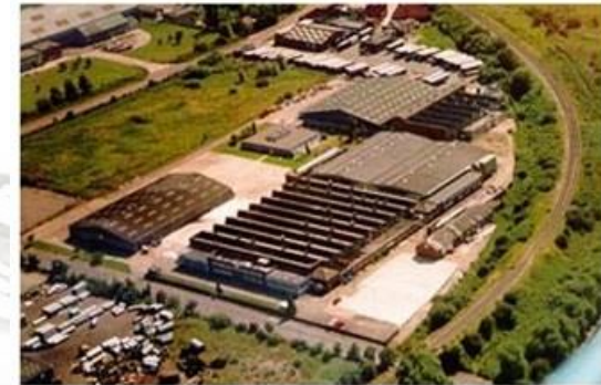
EnerSys Newport Facility Newport, Wales, United Kingdom
